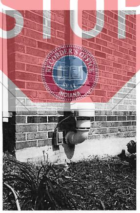
Once the building construction is complete, EVAJO LLC will complete sampling of the newly installed system piping for VOCs by EPA Method TO-15. The data will be reviewed, and a decision made to complete the installation of the sub slab depressurization system.
